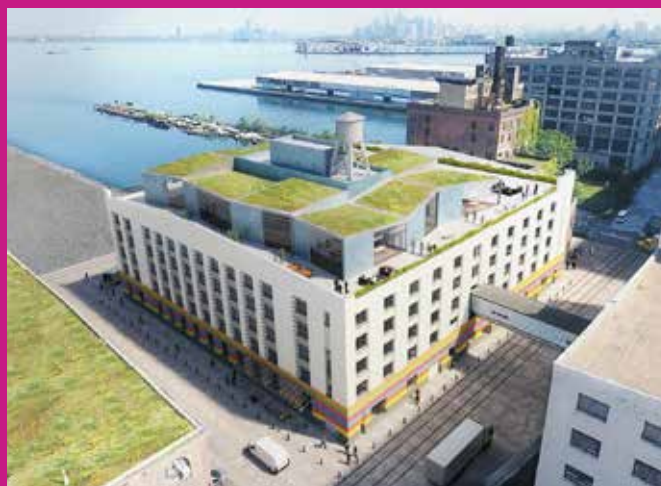
'Made in NY' Campus door WXY
